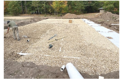
Barnes Park drain field replacement.
